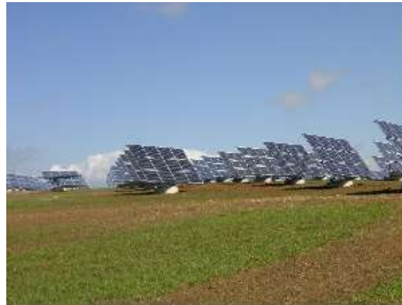
11 MW Germany 2006 Dual axis trackers
