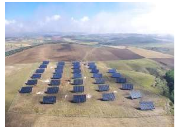
1.1 MW Spain 2008 Single axis trackers
