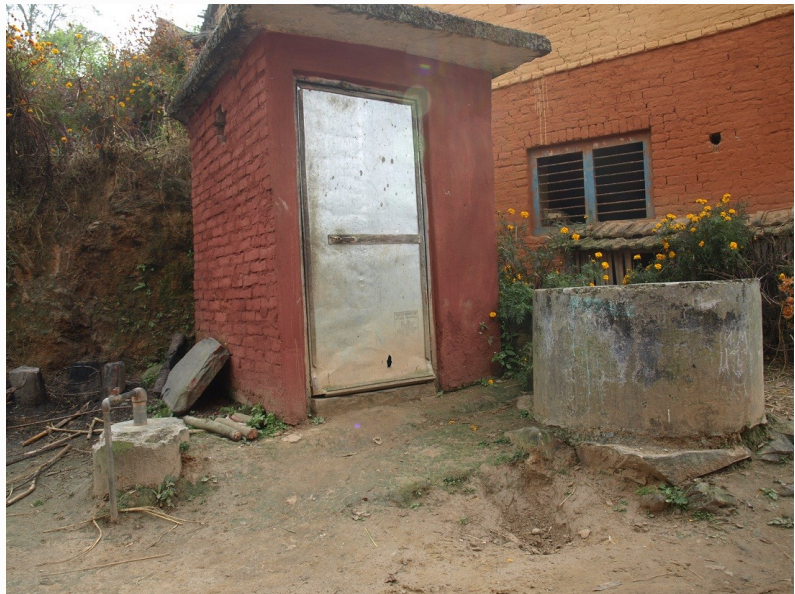
Figure 1: Toilet Attached GGC 2047 Biogas Plant
