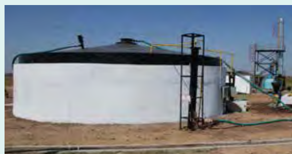
Institutional biogas plant at Muni Seva Ashram, Waghodia.
