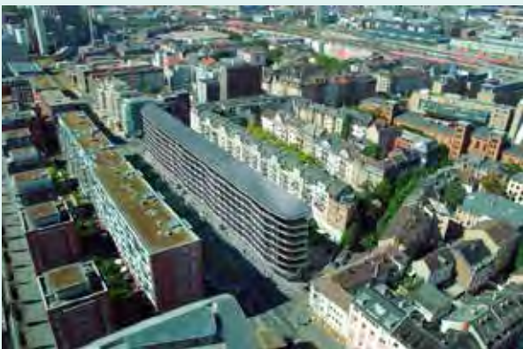
Solar PV on the roof of the "Active House" in Frankfurt.
