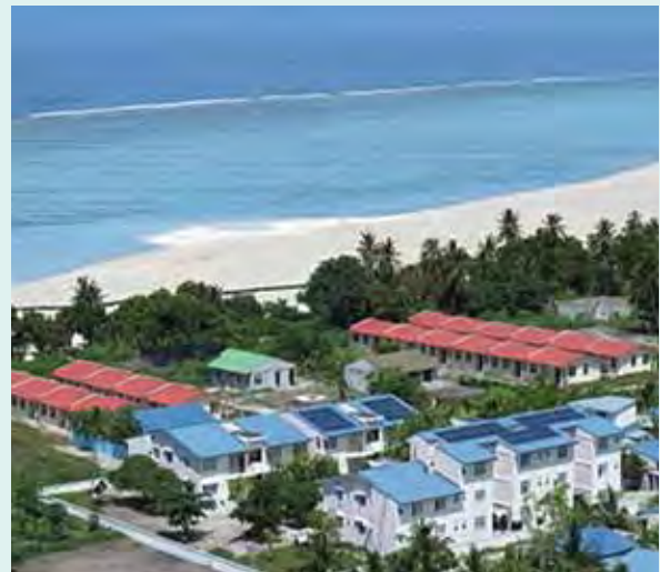
Solar installation on residential buildings on Kudahuvadho Island, Maldives.
