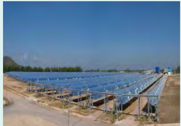
TSE1 – The first commercial solar thermal parabolic trough power plant in the world based on direct steam generation.
