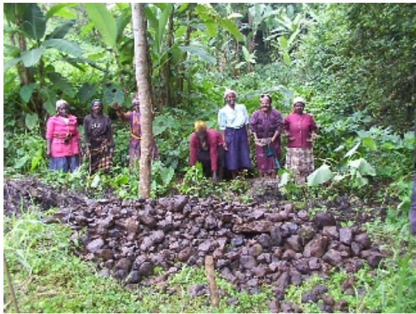
Collecting hardcore for the foundations
