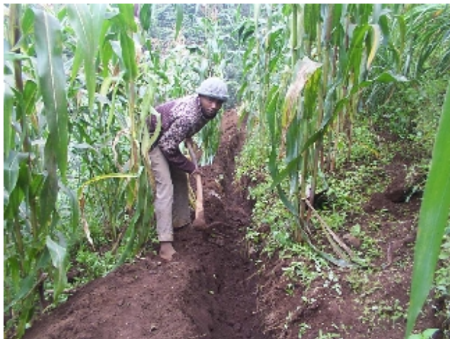
Digging the penstock trench
