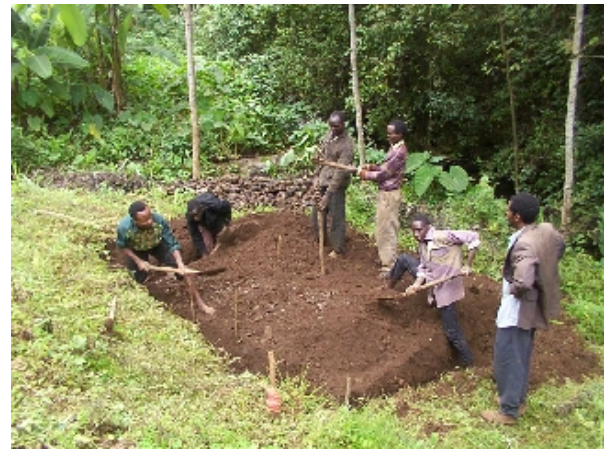
Digging out the footing for the walls.
