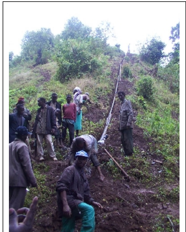
Laying the pipe from the intake to the turbine house.
