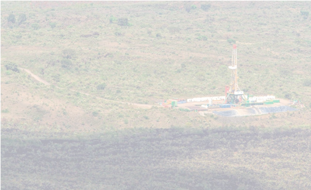
Geothermal power plant in Menengai Crater, Nakuru, Kenya
