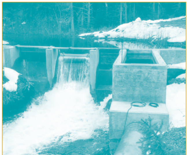
Figure 31. Headwork structure and screen in Morehead Creek, British Columbia (photo courtesy of Thomson and Howe Energy Systems Inc.)
