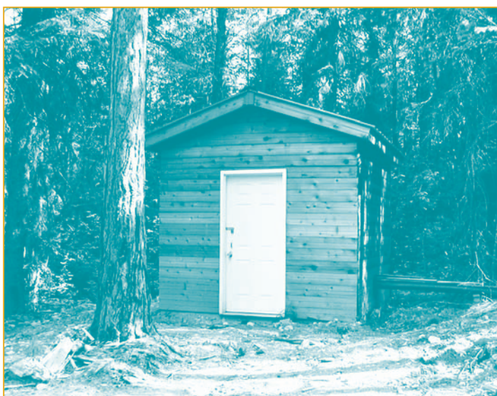
Figure 16. Powerhouse for an 8-kW system (photo courtesy of Thompson and Howe Energy Systems Inc.)
