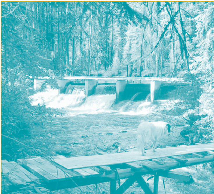
Figure 3. A typical micro-hydropower weir in Cherry Creek, British Columbia
