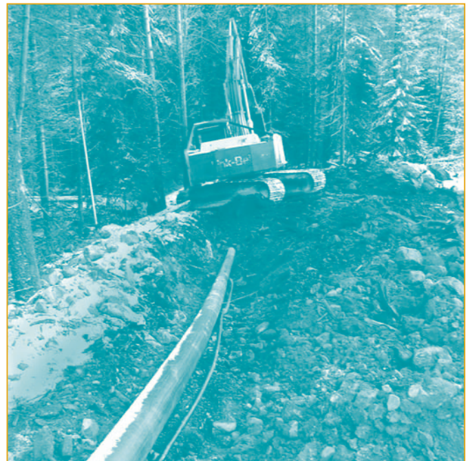
Figure 29. Burying a 20-cm (8-in.) Penstock pipe (photo courtesy of Thomson and Howe Energy Systems Inc.)
