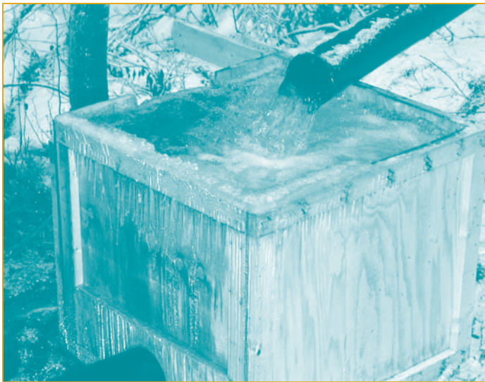
Figure 13. Wooden screen for a 24-kW micro-hydropower system (photo courtesy of Thompson and Howe Energy Systems Inc.)
