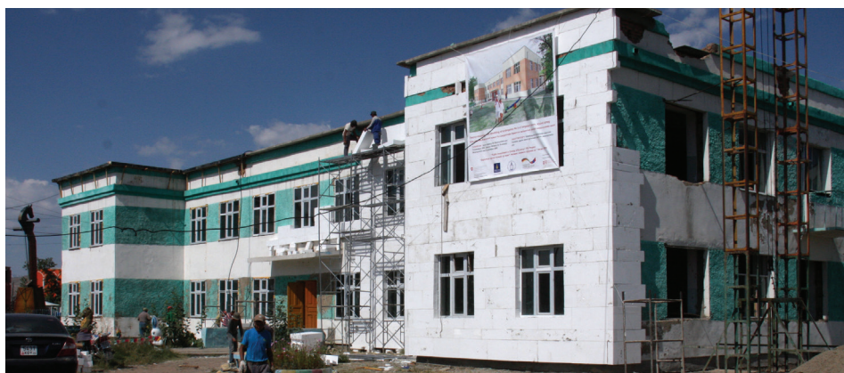
Kindergarten in Khovd under renovation
