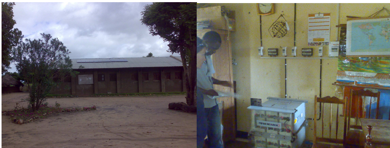
School with Solar electrification
