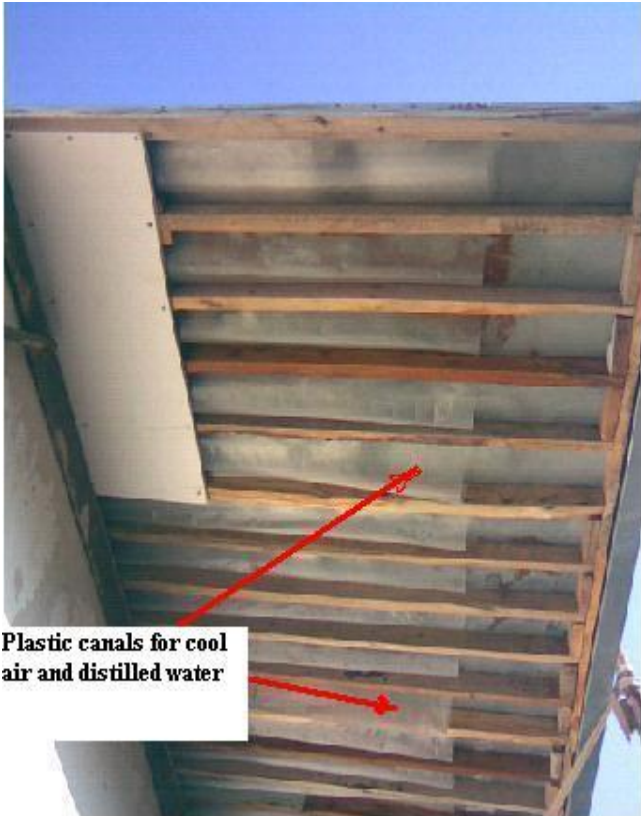
Figure 2: Lower end of the canals for the moisturized air.
