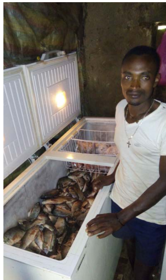
Figure 12: ©Rensys Engineering & Trading PLC-solar mini-grid powered refrigerator being used for income generating activity on Dek Island, Ethiopia.
