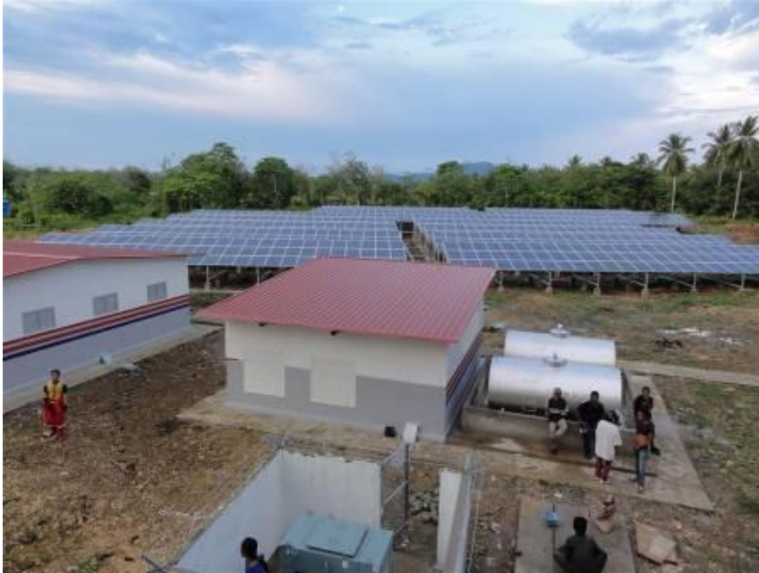
Source: IBC Solar AG
