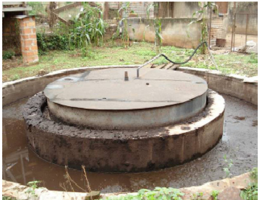
Picture 7 and 8: Examples of floating drum biogas digesters. On the left side, digester made out of poly-ethylene tanks and on the right side constructed with bricks and steel.
