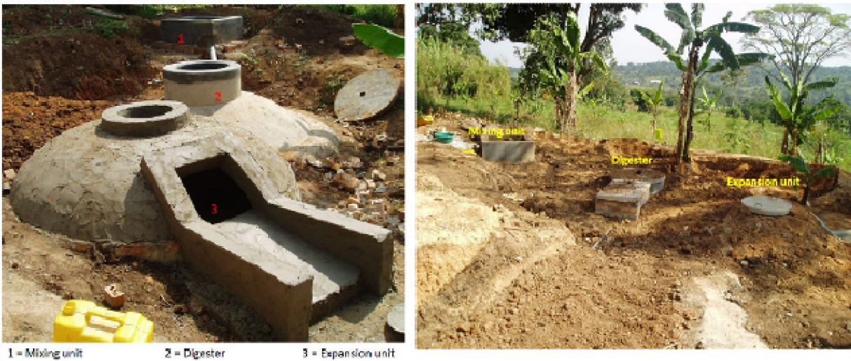
Picture 5 and 6: Fixed dome biogas digester in Buwambo during construction
