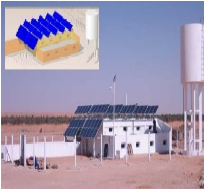
Station de descellement P= 10 Kwc V=15m 3 /j Inv= 540MDT 2006
