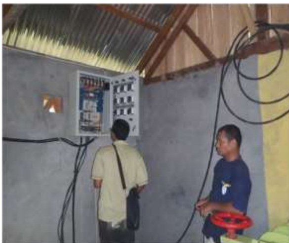
Figure 6-4: Measuring MHP Technical Performance a) meter reading on KPI Survey b) photo of various installed electrical meters installed on the control panel
