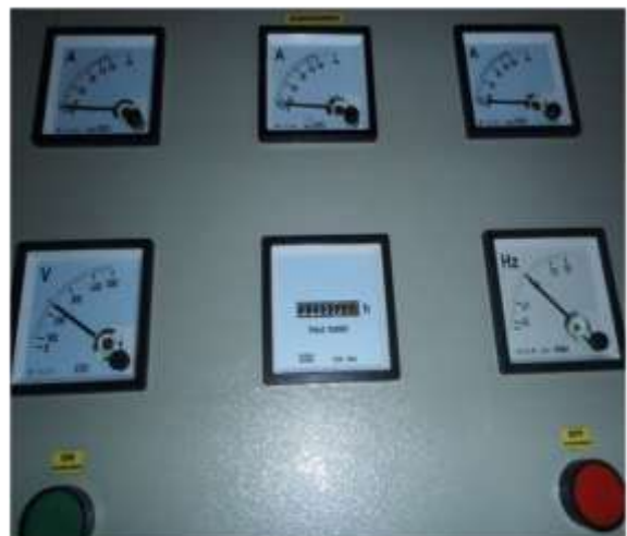
Figure 6-4: Measuring MHP Technical Performance a) meter reading on KPI Survey b) photo of various installed electrical meters installed on the control panel
