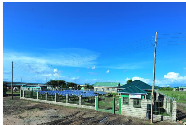
A 40 kW p solar hybrid mini-grid pilot project implemented by GIZ ProSolar in Talek trading centre, Narok County – Kenya.
