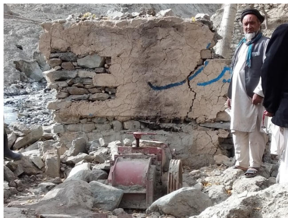
MHP 2011, total flood destruction
