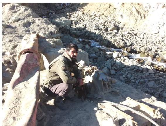
MHP 2013, total flood destruction
