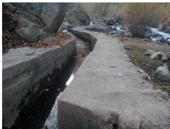
MHP 2017, concrete channel section
