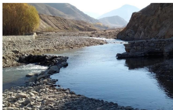
MHP 2103, temporary weir
