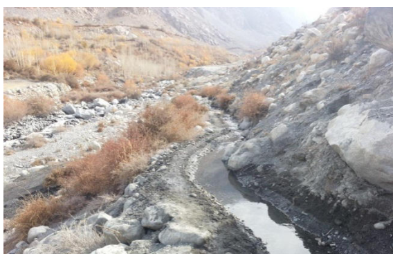
MHP 1085, earthen channel
