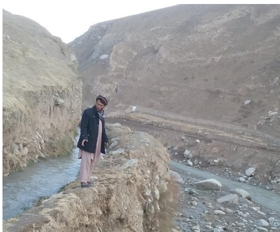
MHP 4120, earthen channel
