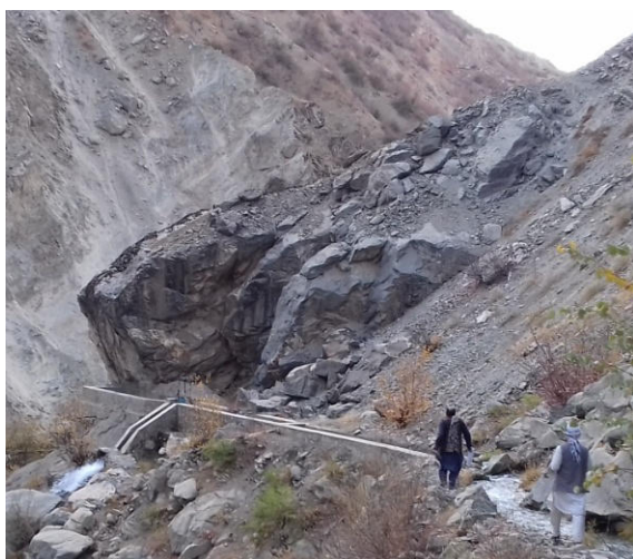
MHP 4048, difficult terrain for MHP construction
