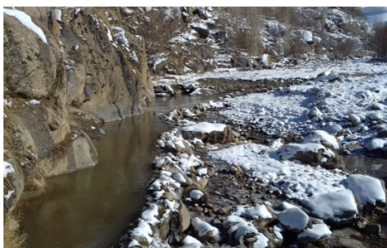
MHP 4122, temporary weir at intake
