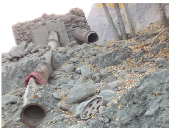
Figure 30 Entirely destroyed MHPs by natural disasters
