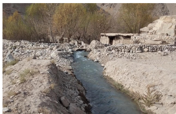
MHP 2100, earthen channel
