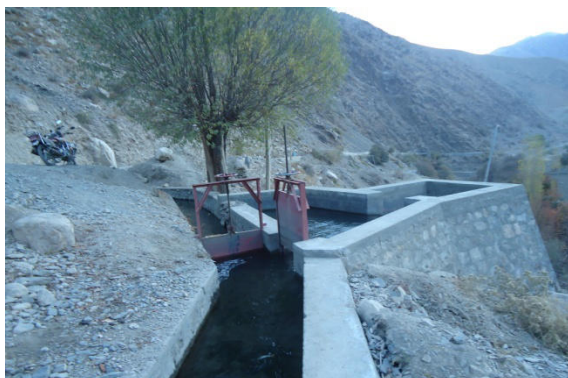
MHP 4079, properly built civil works
