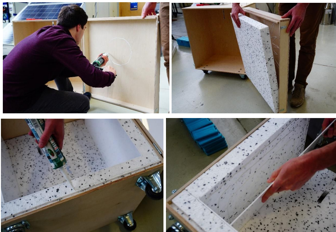
Figure 24: Gluing of the polystyrene insulation and internal acryl glass covering
