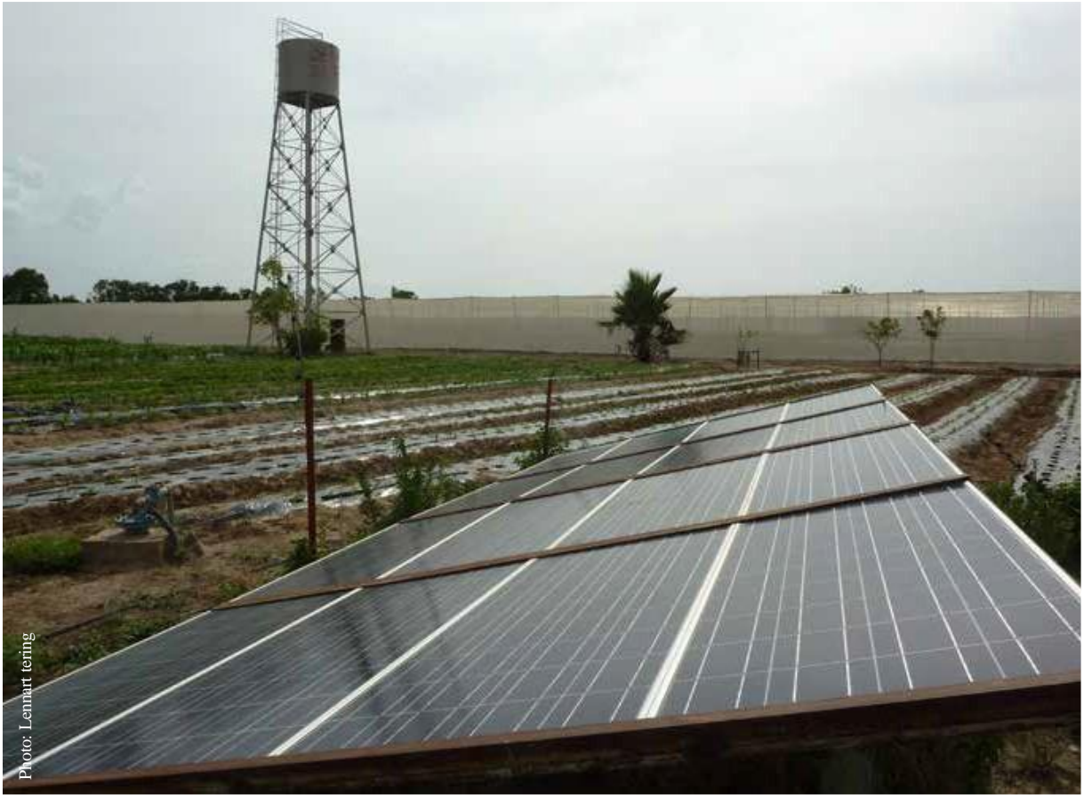
SPIS with an elevated reservoir used for irrigation in- and outside of the greenhouse (Source: Lennart Woltering)
