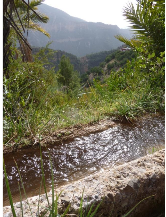
Concrete irrigation canal
