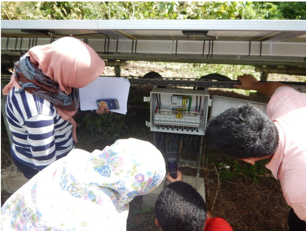
Figure 18 DG NREEC staff are conducting measurement at combiner box
