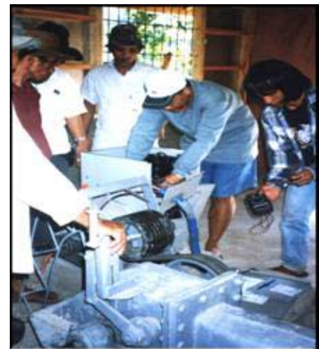
Figure 18. Installation of the alternator
