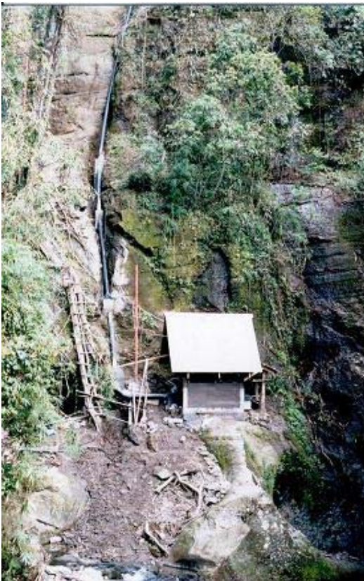
Figure 59. Construction of Lon-oy Powerhouse
