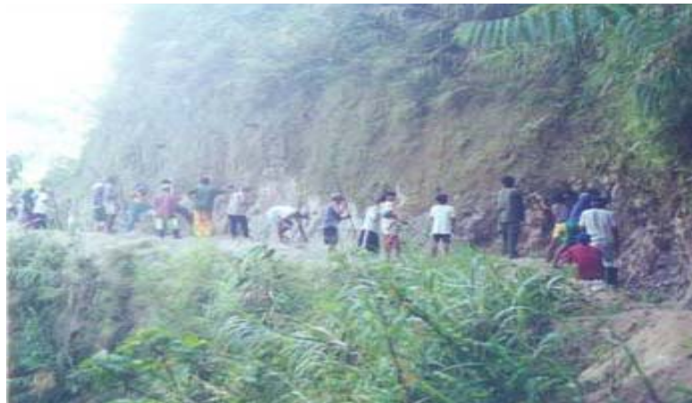
Figure 28. Widening of the irrigation canal cum power canal of the MHP
