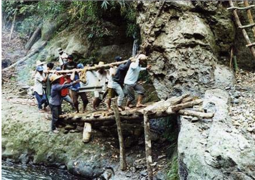
Figure 61. Hauling the turbine to the powerhouse site
