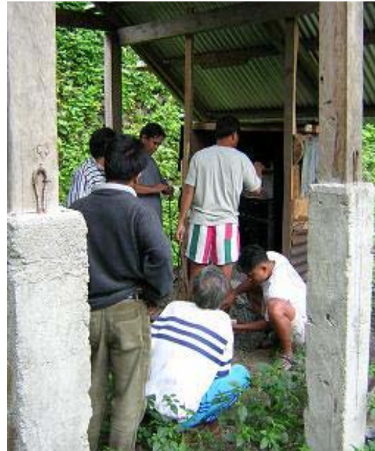
Figure 53. Installation of the sugar cane press
