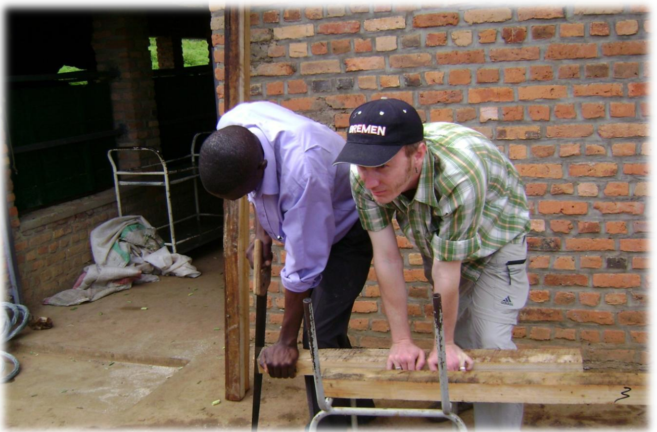
Figure 12: Sawing of the wood for the reservoir suspension construction
