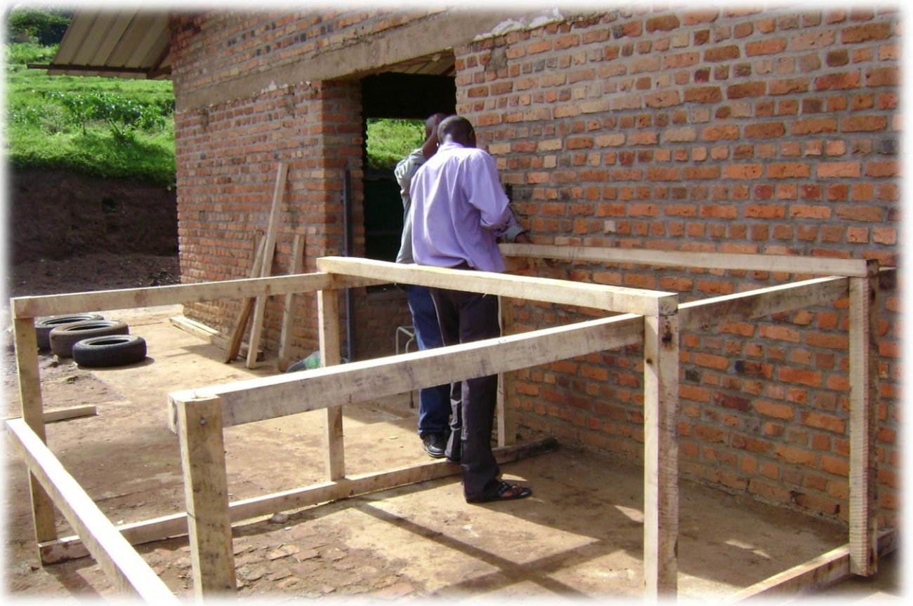
Figure 13: Installation of the reservoir construction
