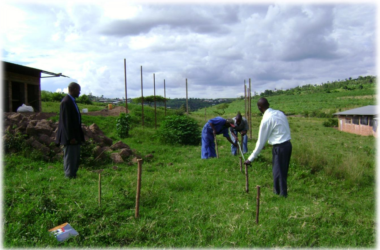
Figure 9: Marking of the trench limits
