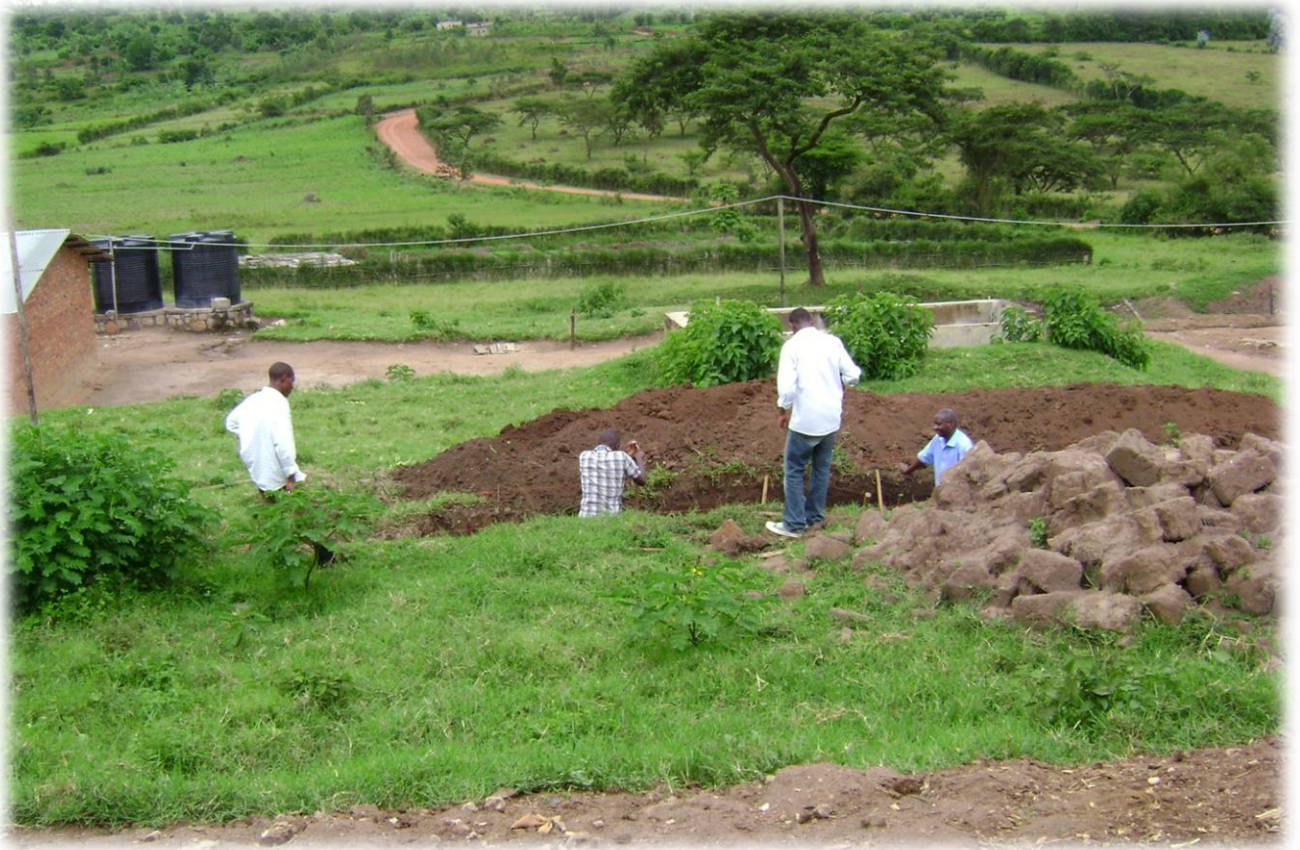
Figure 11: Digging of the trench
