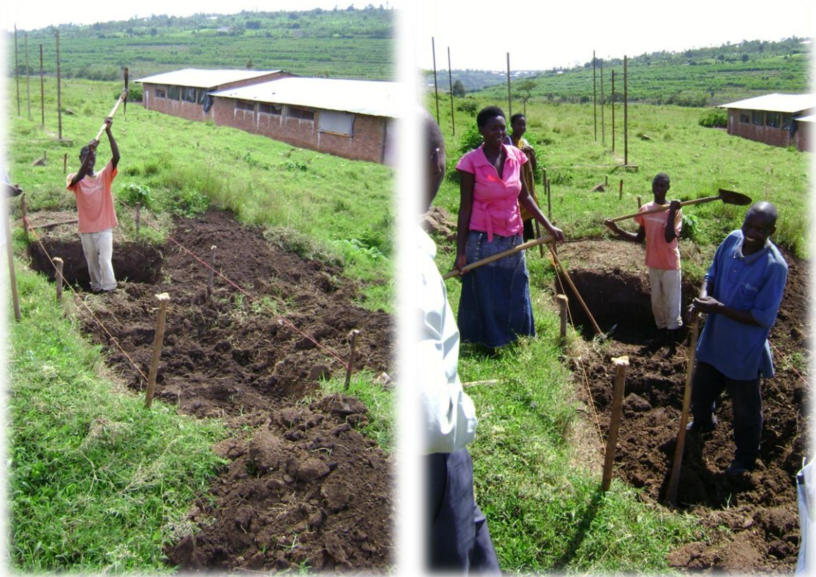
Figure 10: Digging of the trench
