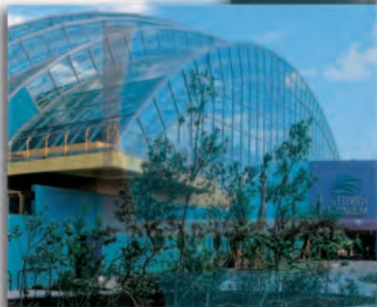
Above: Florida Aquarium Location: Tampa, Florida Architect: HOK, Inc. Tampa, Florida Product: XIR™ Sea Foam Clear
