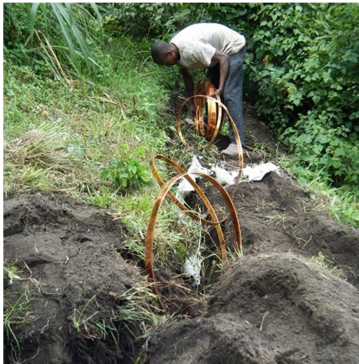
Laying ground electrode through a solid copper band
