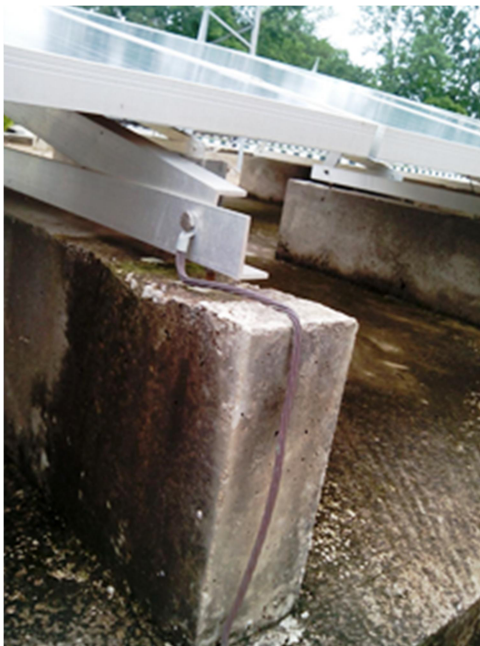
Grounding the metal frame of a solar array
