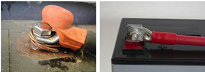
Poor connection (left), good connection (right)
