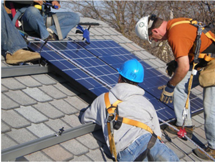
Solar PV installers wearing all required PPE – Courtesy: www.thesolarplanner.com
