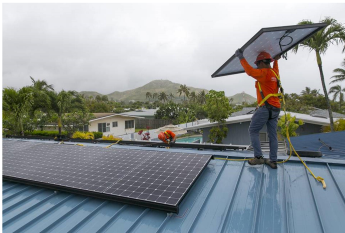
Solar PV installer in Hawaii with fall protection
