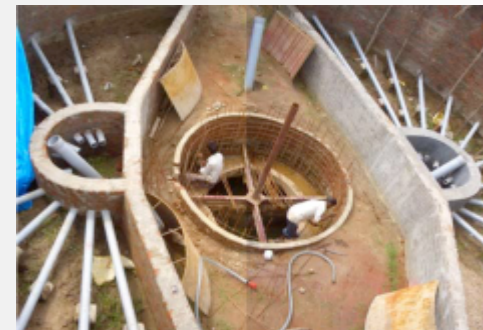
biogasreactor in the center of the building
