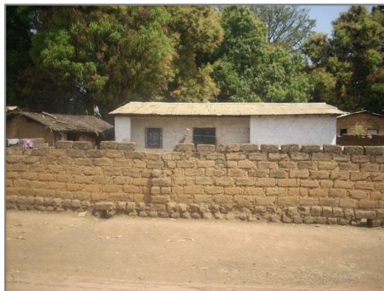
Figure 22 : Standing de type haut, zone nord
