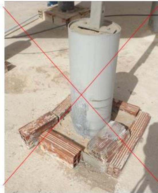
FIGURE 20: EXEMPLE DE DEFATS DE LESTAGE CONSTATES
