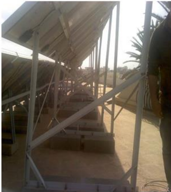
FIGURE 20: EXEMPLE DE DEFATS DE LESTAGE CONSTATES
