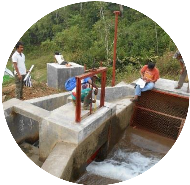
Assessing the civil work of a micro hydro power requires thoroughness and carefulness. (Source: EnDev ID, GIZ)
