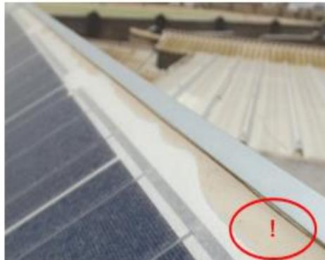
FIGURE 2: DELAMINATION
