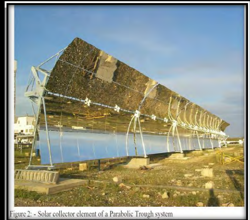
Figure 2: - Solar collector element of a Parabolic Trough system
