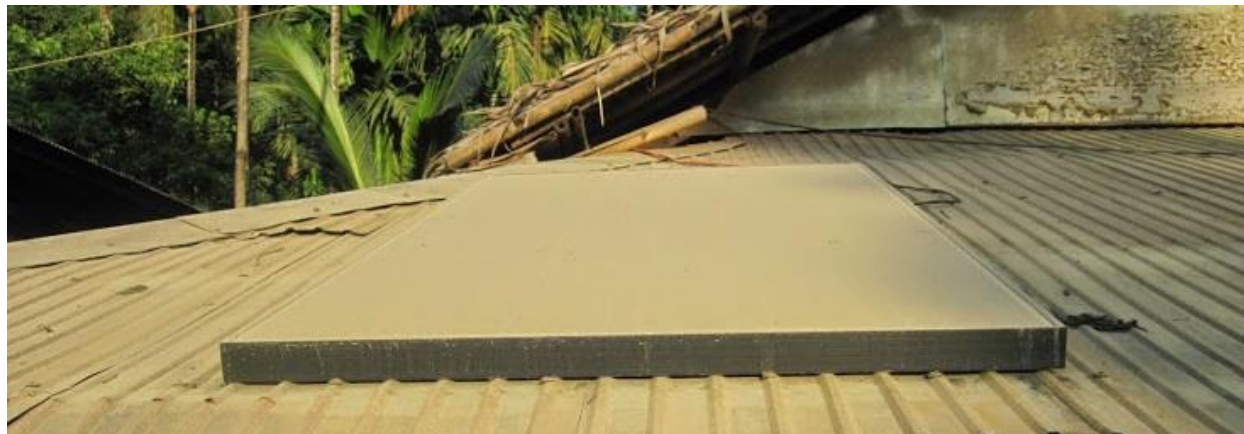
Figure 13: Dusty solar panel on roof
