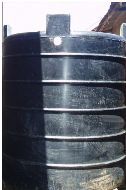
Make a 63mm hole for the OUTLET at the TOP of the tank
