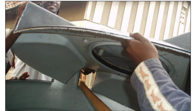
Cut the top off the 1500I DIGESTER tank like this
