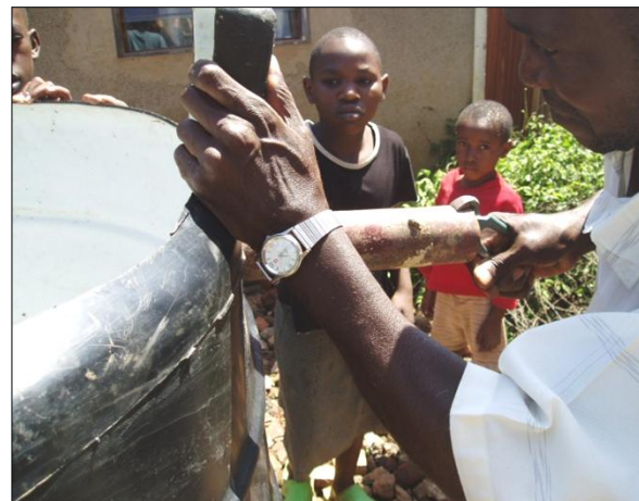
Make a 63mm hole for the OUTLET at the TOP of the tank
