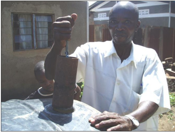
Make a 75mm hole for INLET near the BASE of the tank on the OPPOSITE side to the OUTLET
