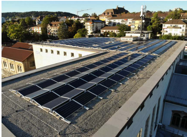
Figure 3: PV array having two different tilt angles.
