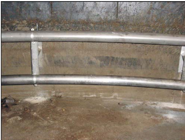
Fig. 6: Inner-lying fermenter heating
