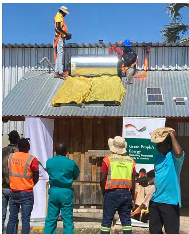
Picture 2: Installation of a solar water heating system
