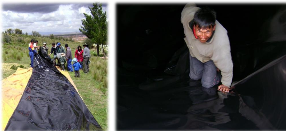
Figure 9: To make the double coat of the polyethylene, somebody has to cross inside the bag and to carry the second bag over the whole length.
