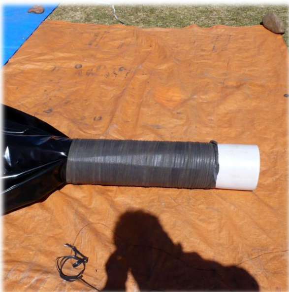
Figure 12: To fix the inlet and outlet pipes with the digester, it is to pick up the lateral of the plastic, to bend them in form of an accordion and then to wind them with the rubber strap.
