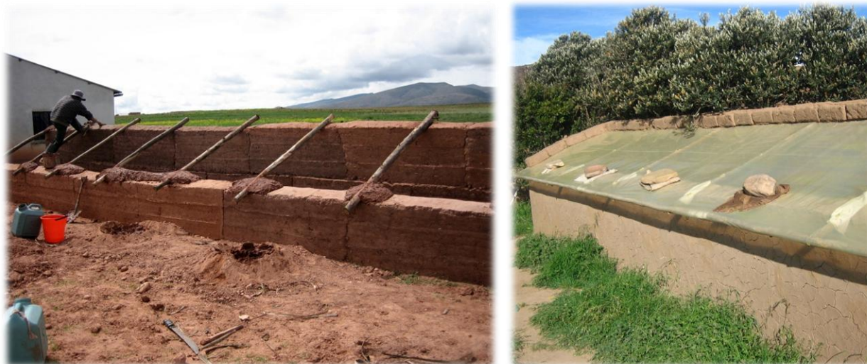
Figure 16: In the high altitude zones a greenhouse is fitted. First it is to fit the bars on the adobe walls and then the greenhouse above the bars.
