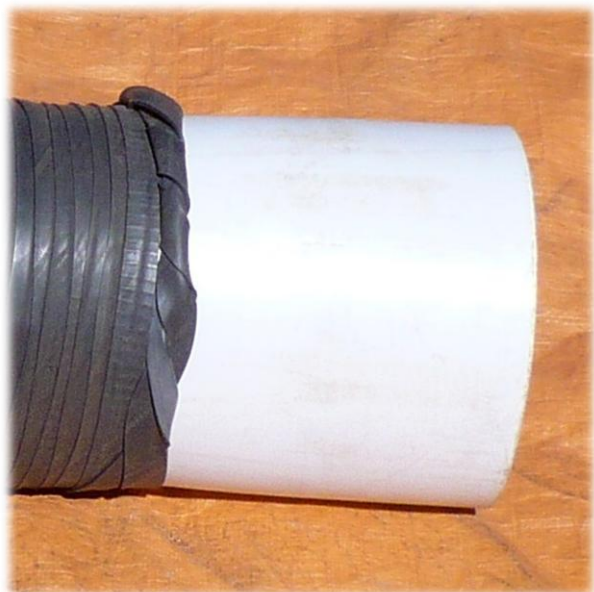
Figure 12: To fix the inlet and outlet pipes with the digester, it is to pick up the lateral of the plastic, to bend them in form of an accordion and then to wind them with the rubber strap.
