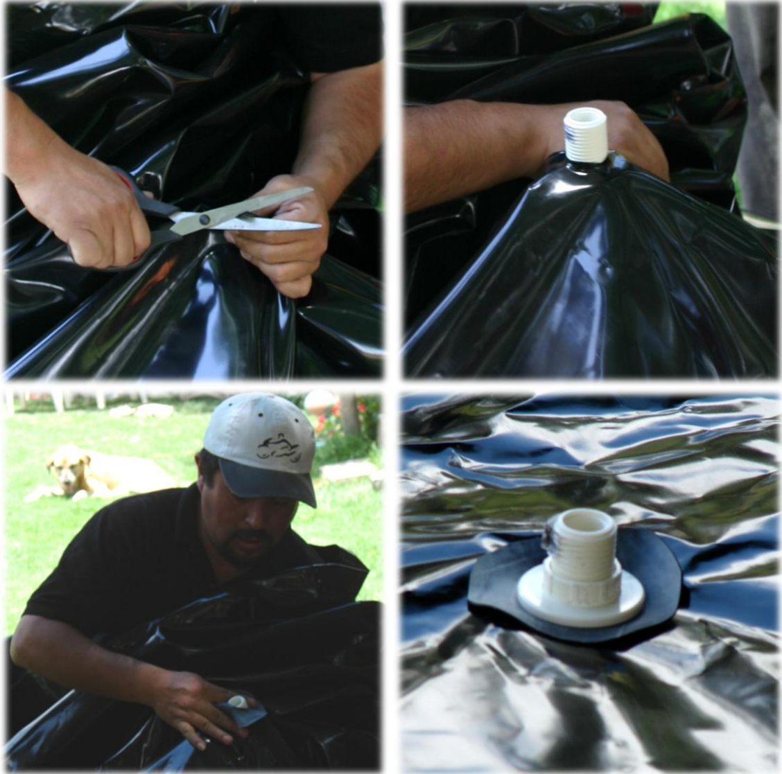
Figure 10: For the mounting of the flange, a cut in the central part of the double coat tube is made. The tightened flange seals the biogas outlet with some rubber pads.
