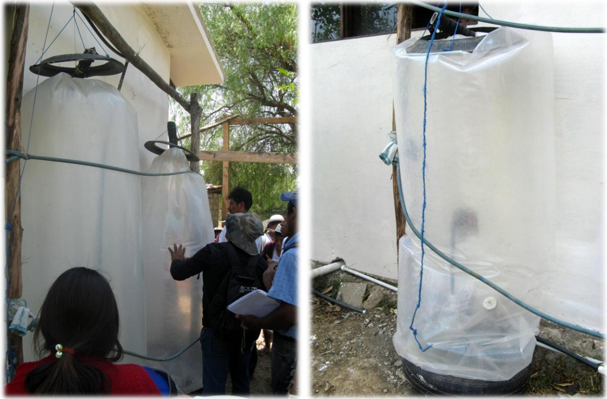
Figure 23: Fixed double reservoir battery with rubber ring for the pressure increasing
