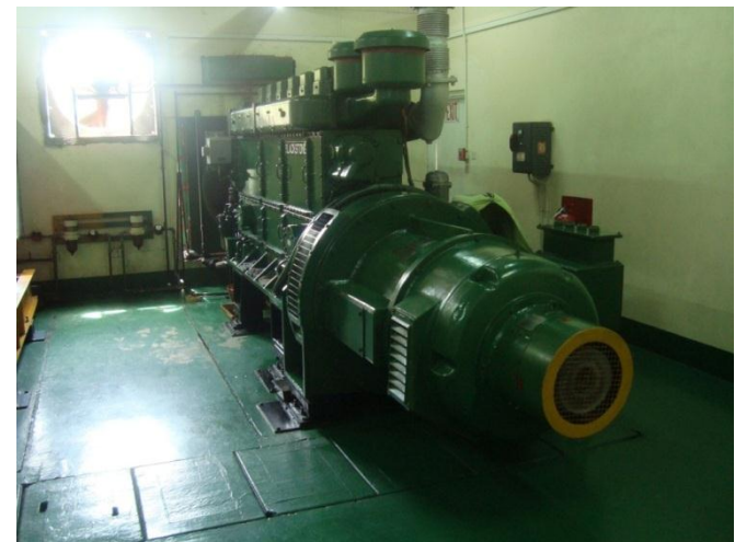
Abb. 4: Diesel GenSet, Lister E 56, Petite Martinique (Blechinger, 2011)
