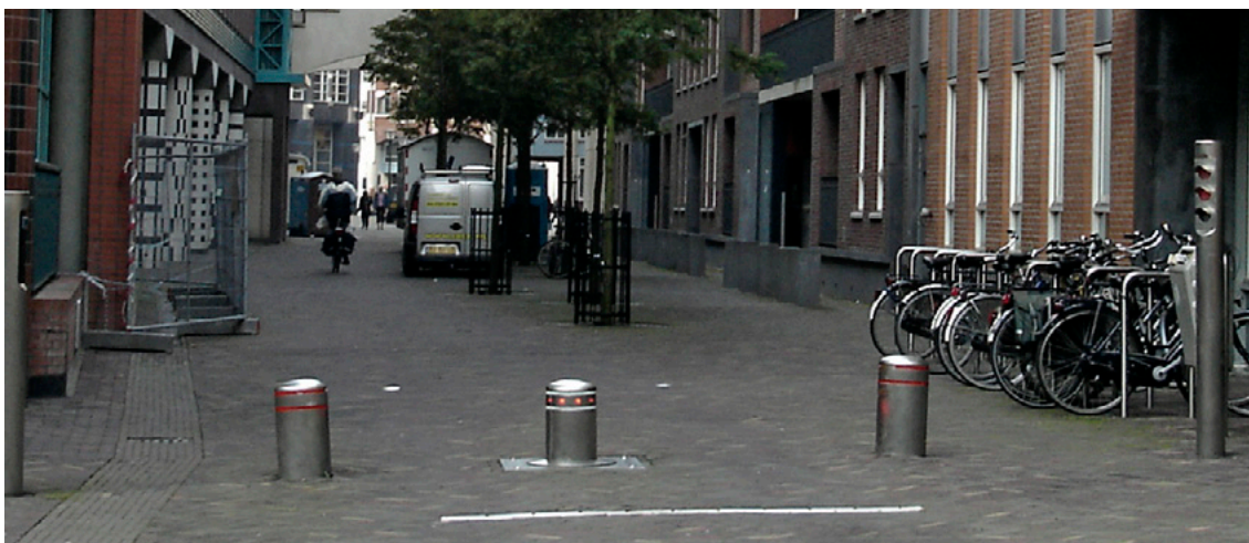
Figure 17 Access control by retractable bollards.
