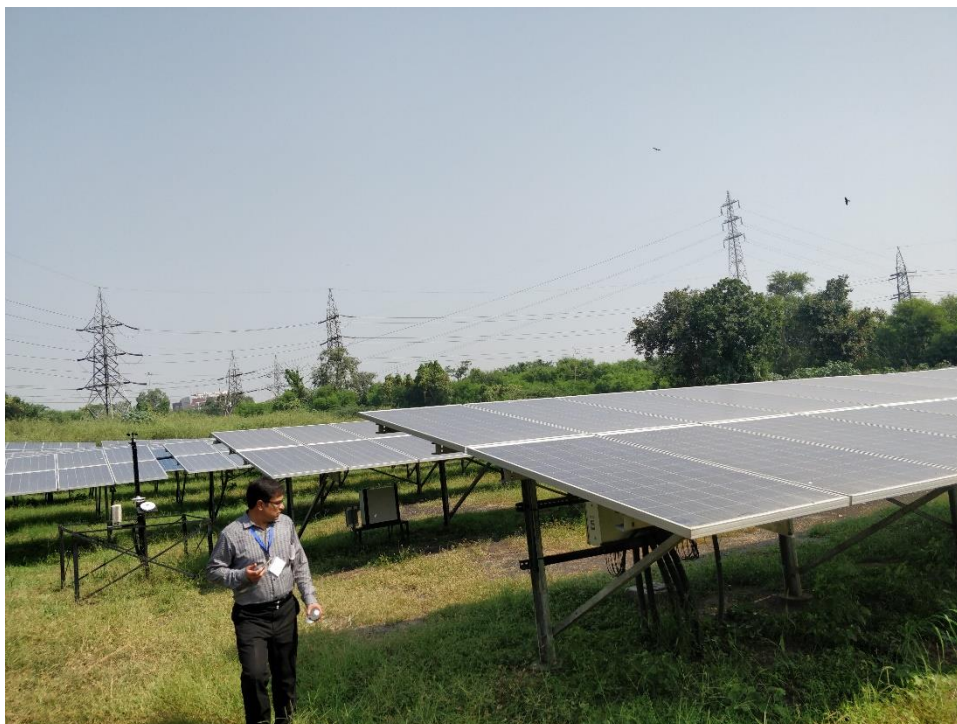
Delegation Visit to Delhi Secretariat Solar Power Plant
