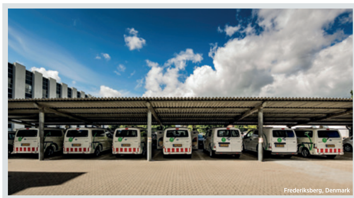
Figure 12 Vehicle-to-grid facilities at Frederiksberg in Denmark
