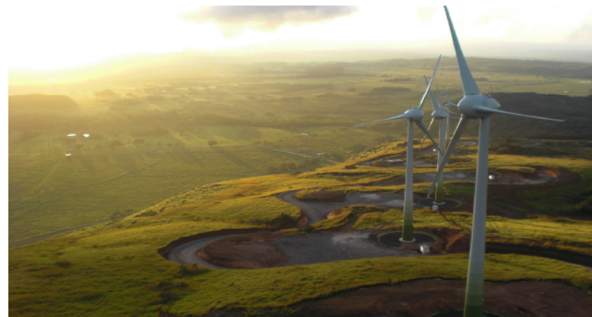
50 MW, Wind farm in Costa Rica
