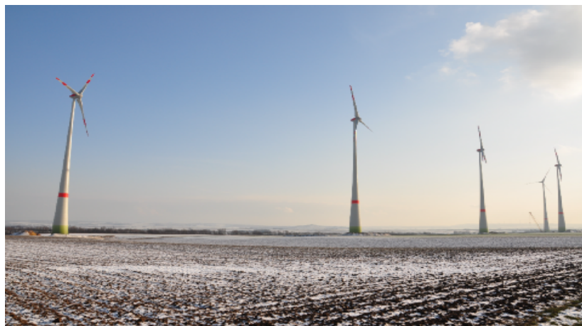
10 MW, Wind farm Wörrstadt
