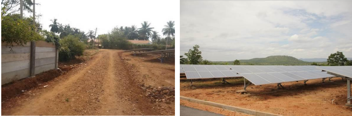
Figure 164: (left) Internal roads; (right) Drainage system
