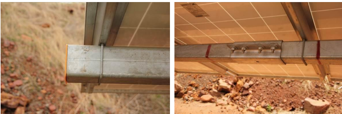
Figure 125: Good surface status of the tracker structure
