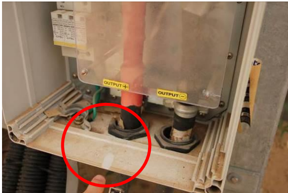
Figure 91: Dust inside the combiner boxes
