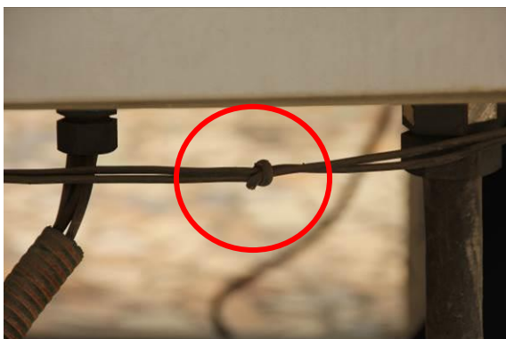
Figure 33: Low bending radius in the string cables
