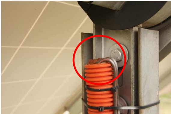
Figure 136: Sealing of the cable ducts
