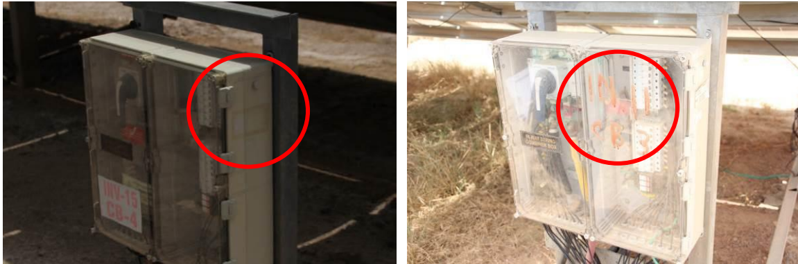
Figure 63: Non-durable labelling of the DC combiner boxes
