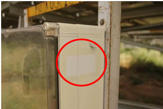
Figure 92: (left) Missing datasheet; (right) Combiner box labelling
