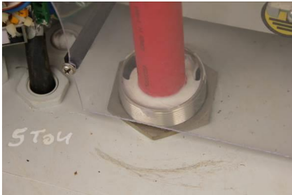
Figure 127: Sealing of the cable glands inside the DC combiner boxes
