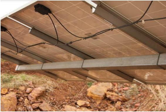
Figure 123: Fixation of the modules to the tracker
