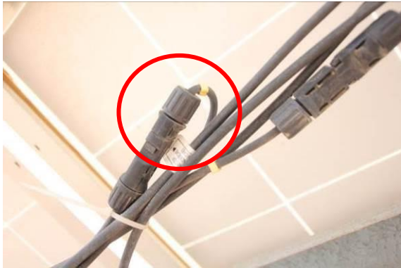
Figure 68: Low bending radius of the string cables
