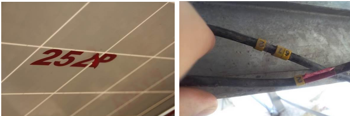
Figure 30: Non-durable string cable labelling
