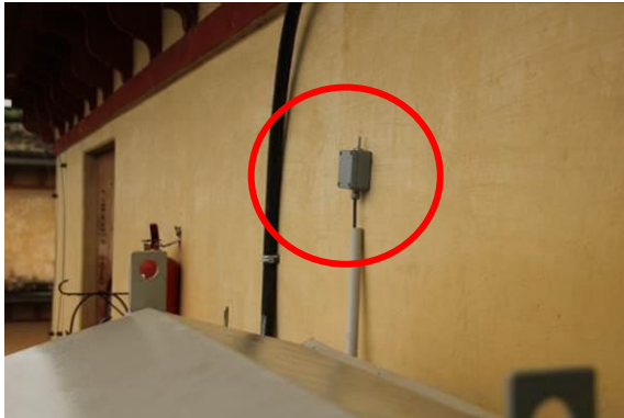
Figure 51: Ambient temperature sensor
