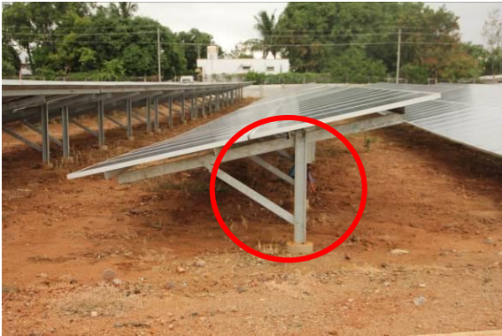
Figure 153: Missing labelling of the module rows
