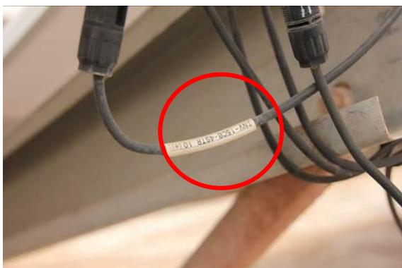
Figure 65: Non-durable string cable labelling
