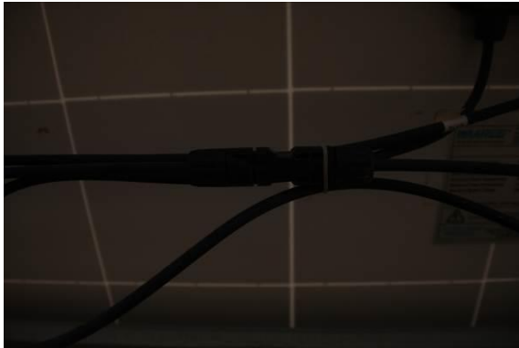
Figure 66: MC connectors
