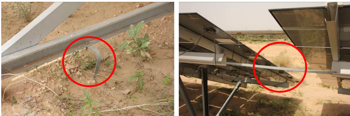
Figure 100: Equipotential bonding system
