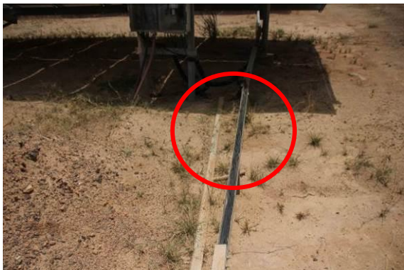
Figure 69: String cables not protected against UV radiation
