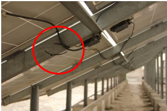
Figure 32: String cables not properly fixed due to degraded cable ties
