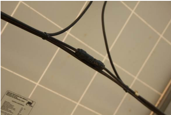
Figure 133: MC4 connectors
