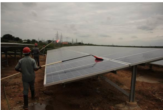
Figure 178: (left) Module cleaning team; (right) Module cleaning device
