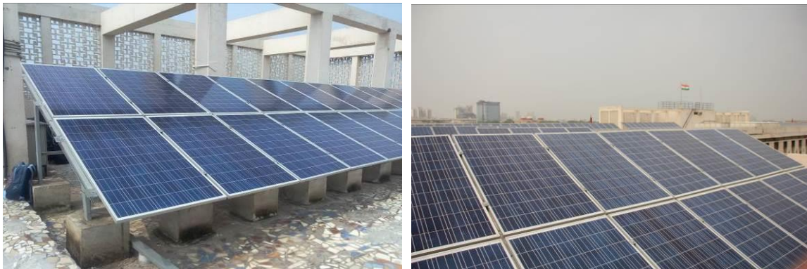
Figure 39: PV modules installed onsite
