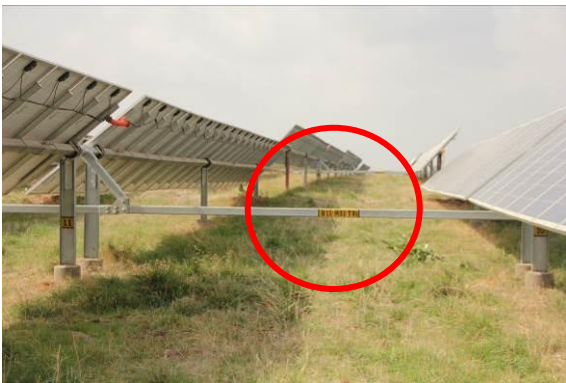
Figure 124: Labelling of the trackers
