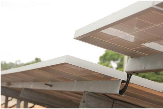
Figure 151: Height differences between the mounting tables in E-W direction
