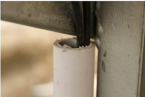
Figure 49: Cable pipes used for routing the string cables
