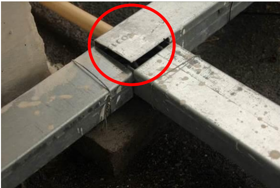
Figure 48: Non sealed cable conduits
