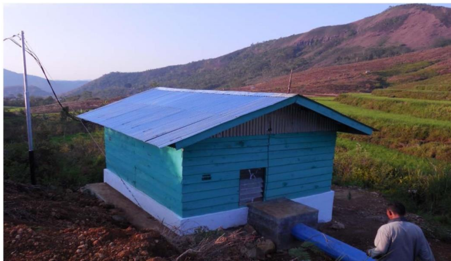
Photo 5: Turbine House of KSU Mute Lestari
