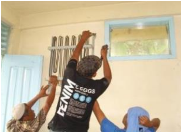
Figure 9 ELC installation in Paninggiran Bawah, West Sumatra
