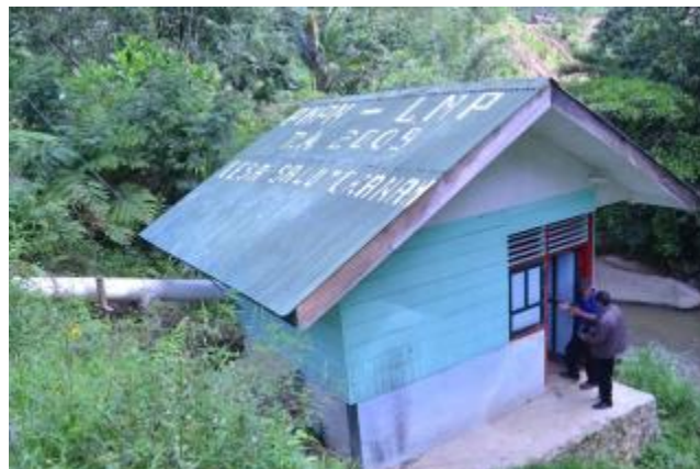
Figure 16 MHP powerhouse in Salumokanan, West Sulawesi
