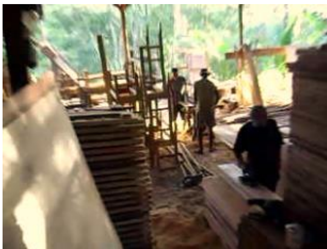
Figure 8 Carpentry in Sungai Keruh, West Sumatra
