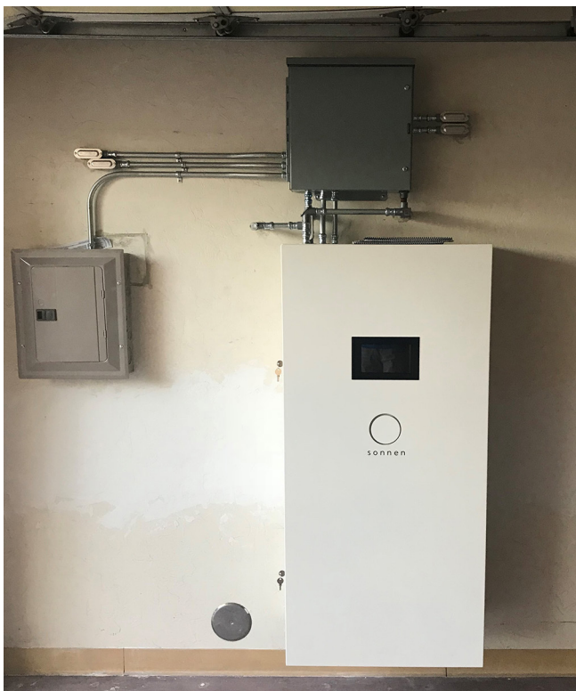
Figure 6 – Example battery energy storage system (indoor) installation
