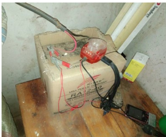
Figure 7. Mix and Match solar system with improper installation.
